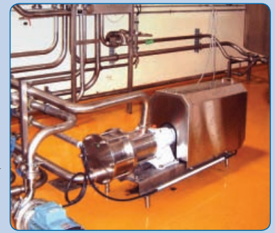
Mouvex C-Series C18i Eccentric Disc Pump.
